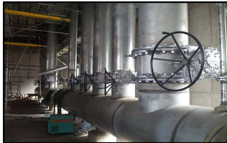
HYUNDAI STEEL BLAST FURNANCE & COG PHASE III FABRICATED TYPE BUTTERFLY VALVE
